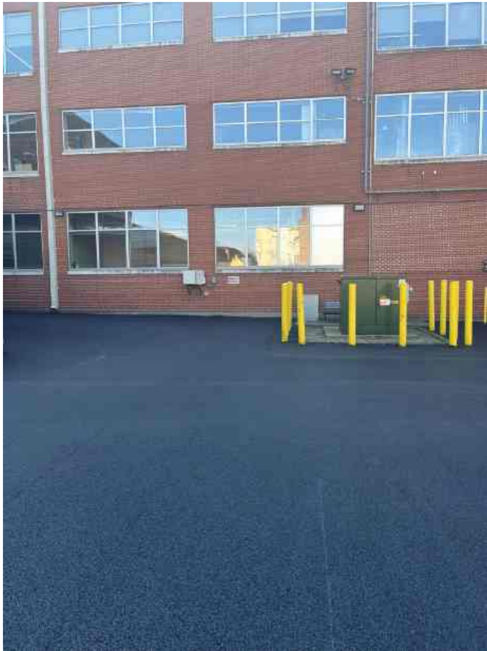
Main Electric Room and E-Bike Locker location
